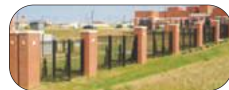
Shown above is another stretch of the fenceline. Unseen are the massive footers which anchor the fence. These were backfilled with dirt and are not visible. (Hercules Fence photos)
