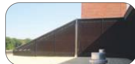
Above, Sentex SL580 operators power the four slide gates on the project. Shown below is a portion of the 579 linear feet of 16-foot-high mini-mesh chain link which was installed on the roofs of three of the buildings to keep birds out.
