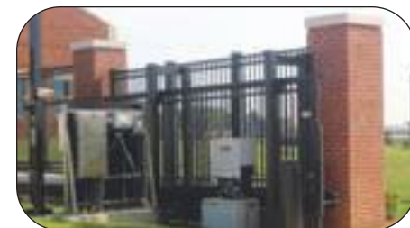
Above, Sentex SL580 operators power the four slide gates on the project. Shown below is a portion of the 579 linear feet of 16-foot-high mini-mesh chain link which was installed on the roofs of three of the buildings to keep birds out.
